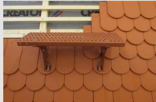
Walking grids, ladders and other accessories of the CREATON system shall not be considered as an anchoring point for safety harnesses.
