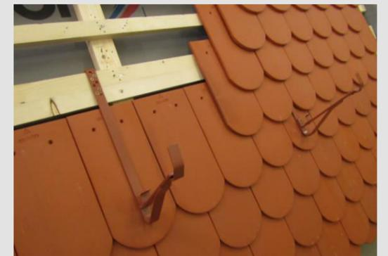
The most suitable place for the linear snow guard is the 2nd row of tiles from the eave in case of single covering and the 3rd row in case of double covering.
