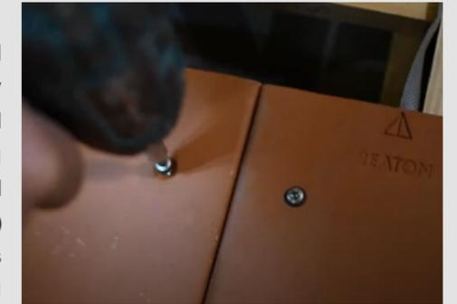
This additional fastening must be carried out for each tile along the listed edges (edge zones) as well as for the fastening of each ridge tile (eg. ridge clip)!
