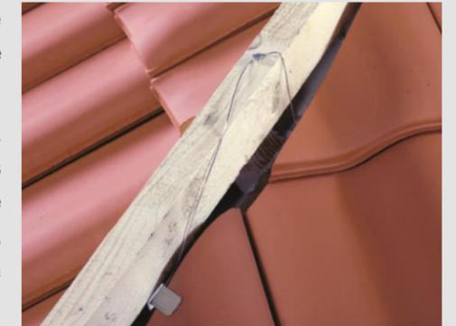
Along the hips and valleys, the cutted tiles can be fixed with a wire. A specially developed product for this purpose is the "Stainless steel clip with wire for cutted tiles", which can be found in the system accessories (see product data sheets) group. In this case, there is no need for a new hole in the tile (so no screw with a sealing head is needed).
